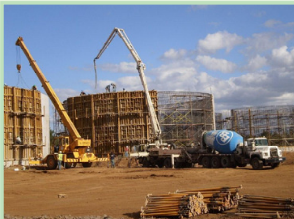
Figure 3: Construction of concrete digesters in typical biogas plant
