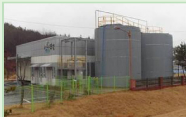
Figure 13: Bousung Biogas Plant 12
