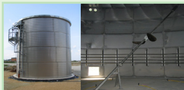
Figure 12: Frankfurt Hahn Airport's co-generation plant showing a pre storage tank (top left), external view of the plant (bottom) and inside of a tank (top right) 11
