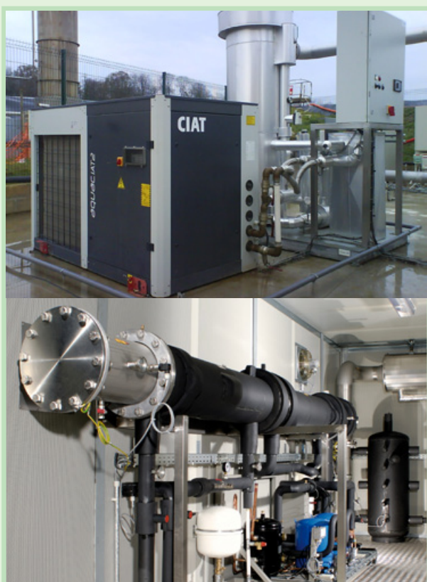
Figure 9: Examples of biogas dehumidifier systems 8
