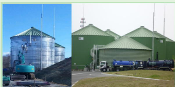
Figure 14: Stainless steel digester tanks at the Shinko Bio Arc 13
