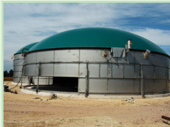
Figure 5: Construction of a stainless steel digester tank 4
