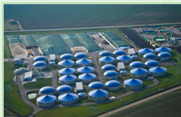
Figure 10: Aerial view of the Saxony-Anhalt biogas plant 9
